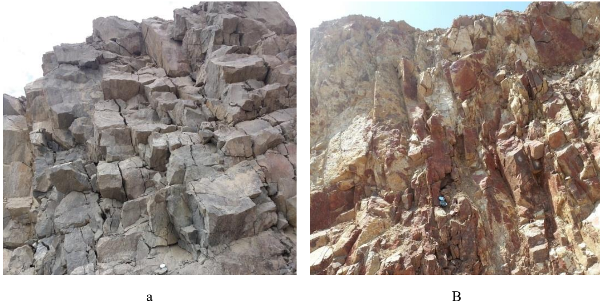
Fig. 5. a) View of a joint located at level of 2250 with a slope of 70 degrees, extension 25, in the direction of slope 295, which is severely crushed. b) View of a joint located at the level of 2287.5 with a slope of 80 degrees, extension 150, direction of the slope of 240 and an average opening of about 1-2 cm.
