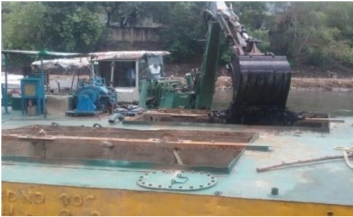
Fig. 1 (a). Dredging work at Najafgarh Drain.
